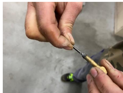
Clean the elbow fitting, e.g. with a drill or a small round file.
